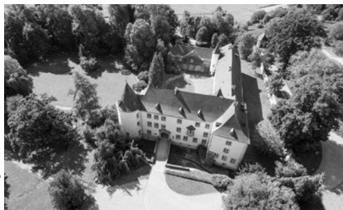
Current situation of the unoccupied castle.
